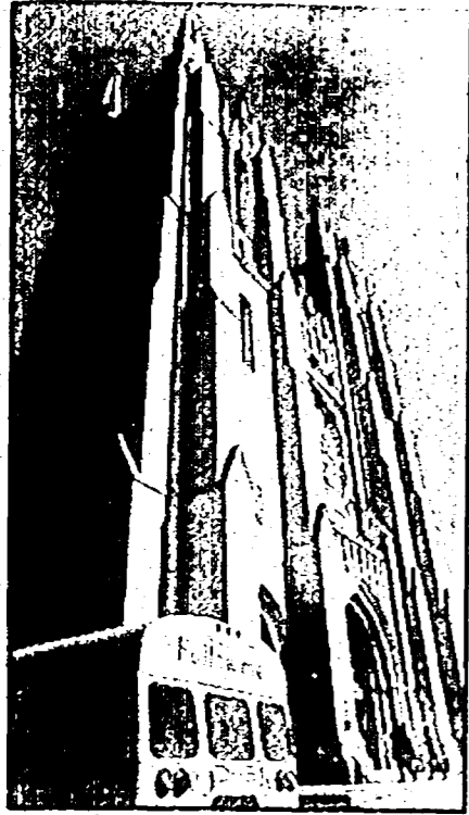
The exterior of Blessed Sacrament Cathedral is an imposing sight.
