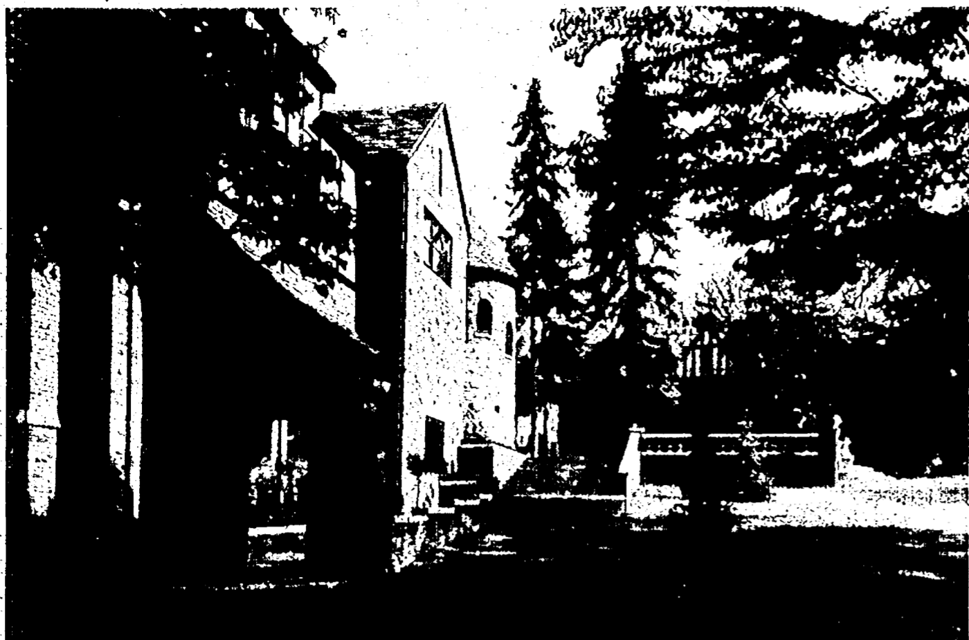
Materials used on the 4,500-square-foot addition to this house built in 1927 were the same as the original. Brick on the addition was hammered and chipped on site to match existing brick.
