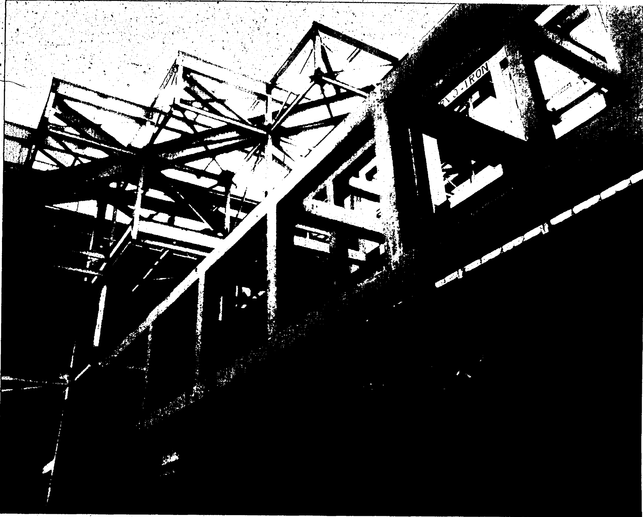
Structural steel detailers produce drawings of every steel connection on commercial buildings. Fabricators make the pieces. Erectors put them
