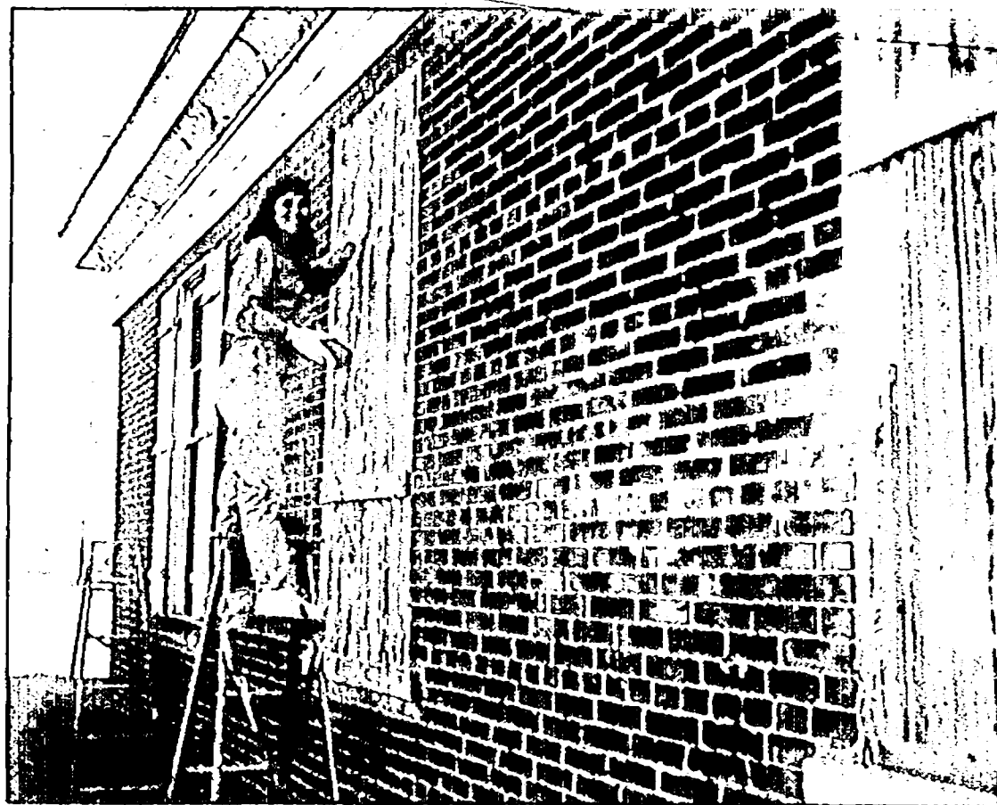
Denise Mehelich scrapes paint off an aging window at the former school.
