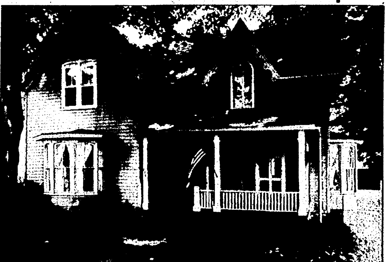
The Frances Barger and William T. Barger Home, built in 1868, reflects Gothic Revival architecture.
