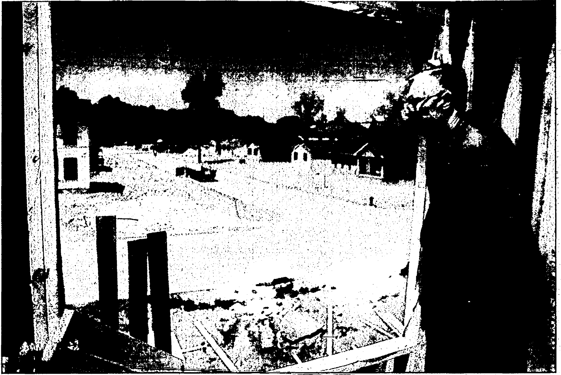
Robert S. Kenning, executive director of Oakland Housing, looks over the River's Edge development from a house under construction in the subdivision.
