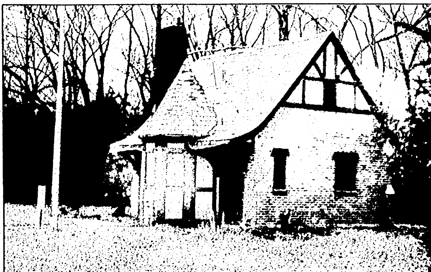
Improving county parks facilities, including long-closed rest rooms is a goal of Friends of Wayne County Parks.
