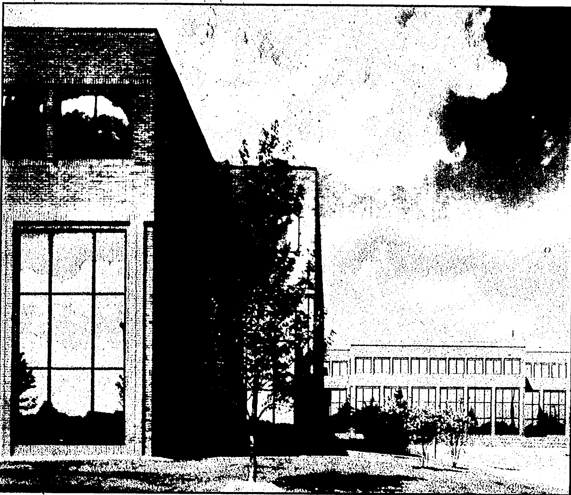
Long Lakes Crossing, Troy, earned Minoru Yamasaki Associates a design award from the Masonry Institute of Michigan. The complex consists of two three-story office buildings, with
