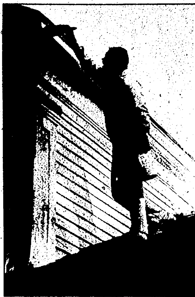
Burt Sloan gets on the roof to paint the building.
