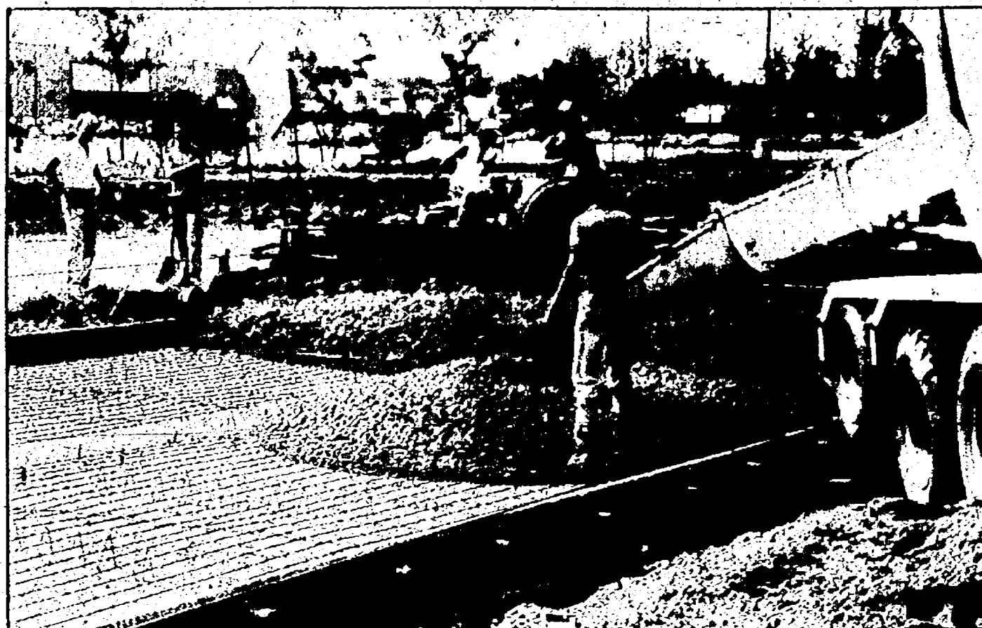
The concrete is smoothed by construction company workers.
