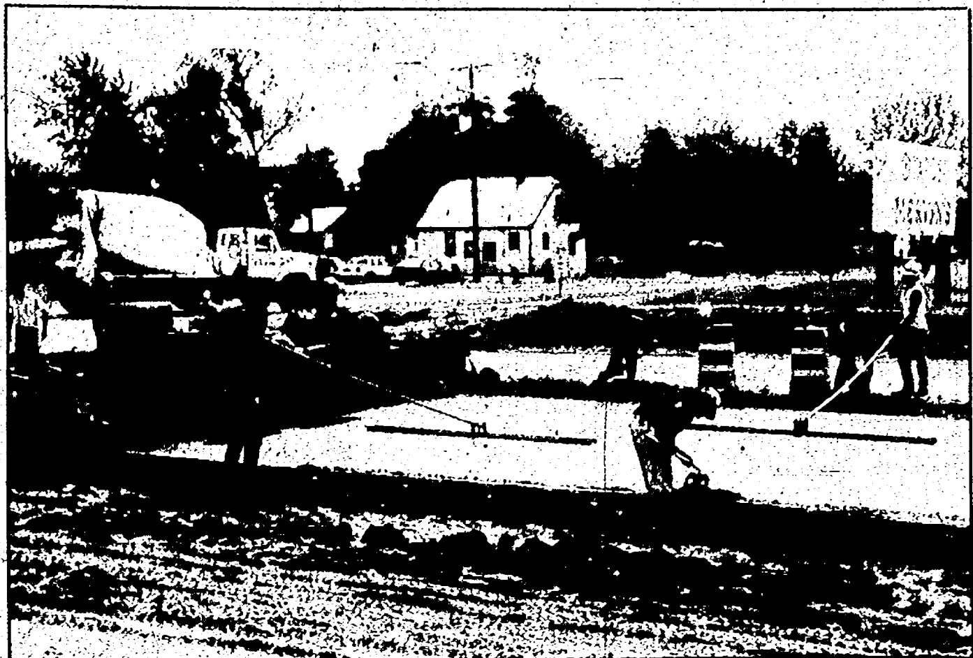
New concrete is poured for the Warren Road widening, expected to be completed in two months.
