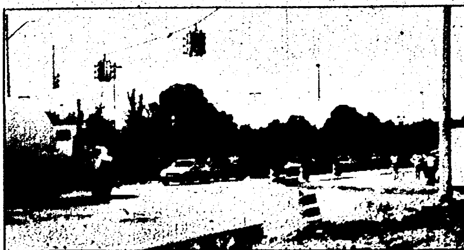
Traffic snakes along Warren Road during the widening construction.
