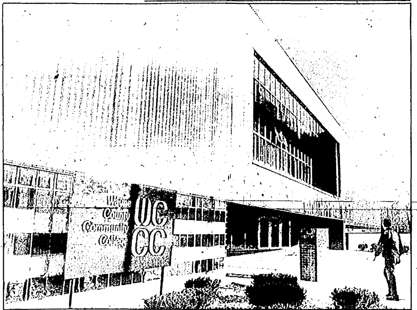
The western campus of Wayne County Community College, in Belleville, provides college courses for over 800 students. The branch wants to broaden its appeal, but its location remains controversial.
