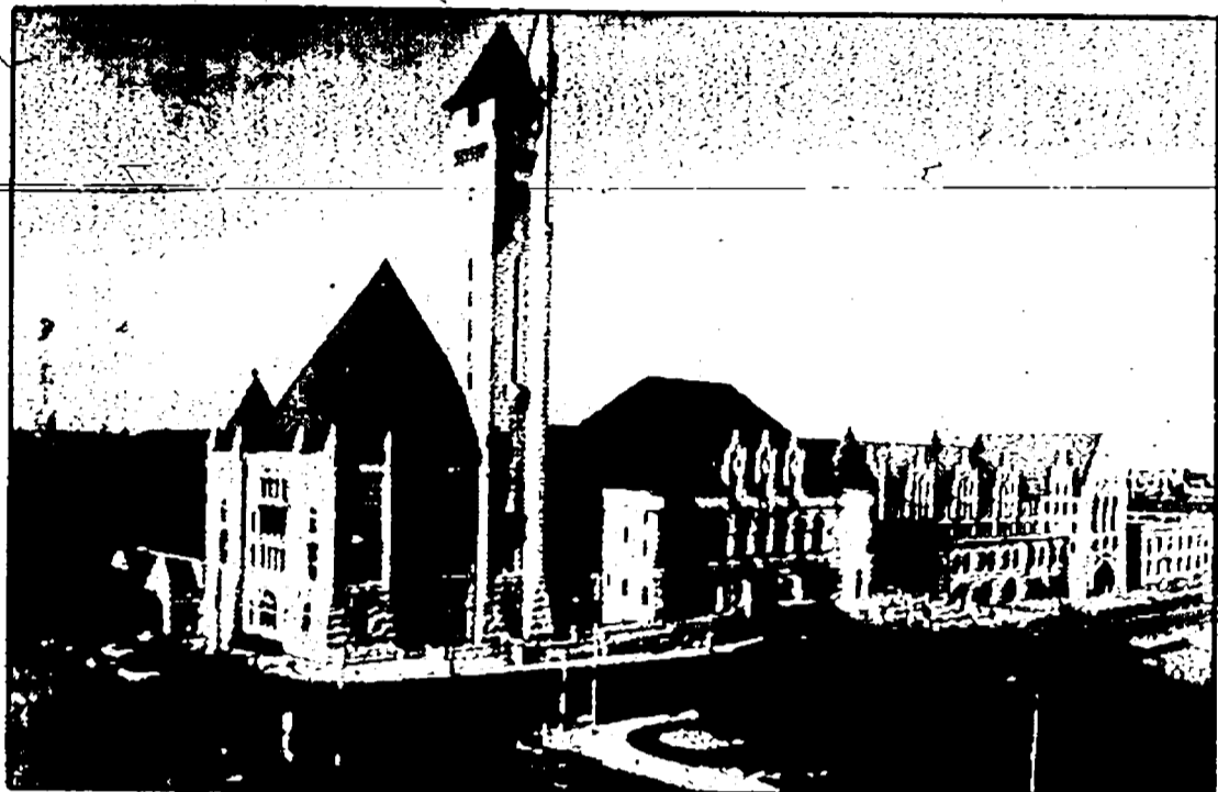
Exterior view of the St. Louis Union Station undergoing renovation. The photo will be part of the Smithsonian exhibition at the Builders Show.
