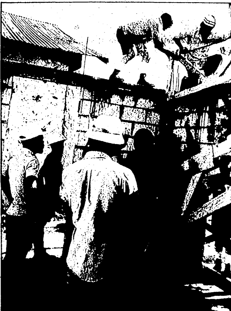
The Haiti work team raises the roof rafters on lay pastor's house.
