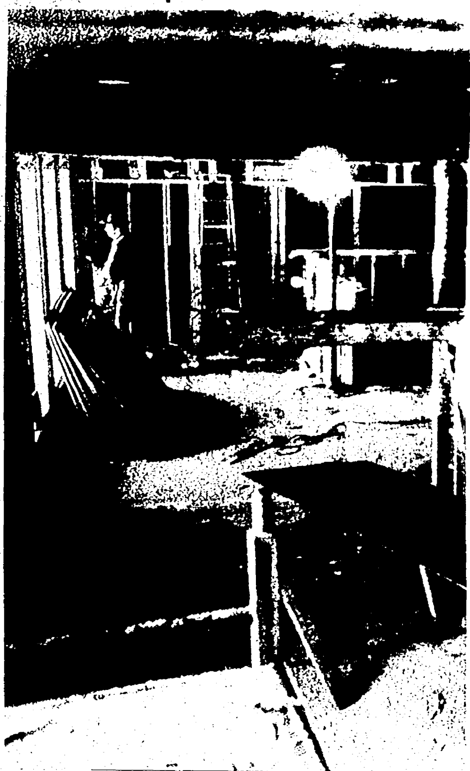
A worker takes a break to check on the wintry weather while work continues on the interior of the former restaurant.
