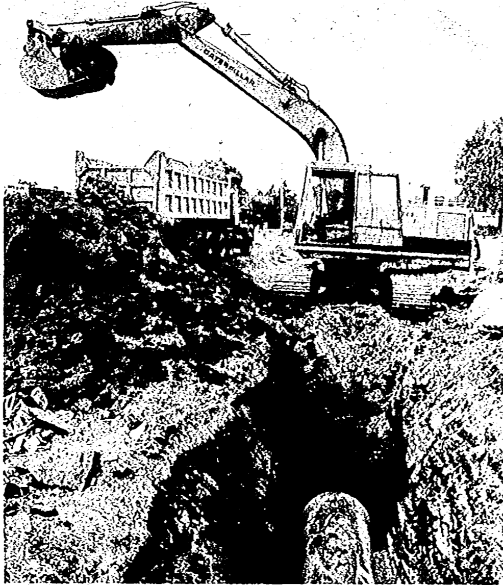
A large steel shovel moves into action, installing new storm sewers on Warren Road between Middlebelt and Inkster. The project is one of three which will total $6.3 million.
