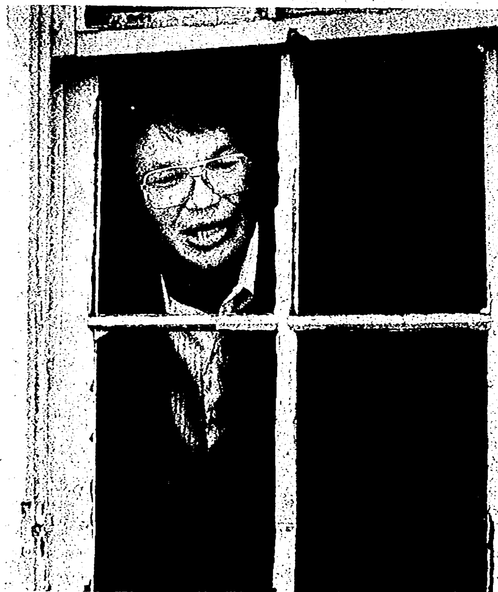
Leon Hanson, a building trades instructor, peers through a broken window pane of the Rowe House, which his students will begin to restore under an agreement with the city.
