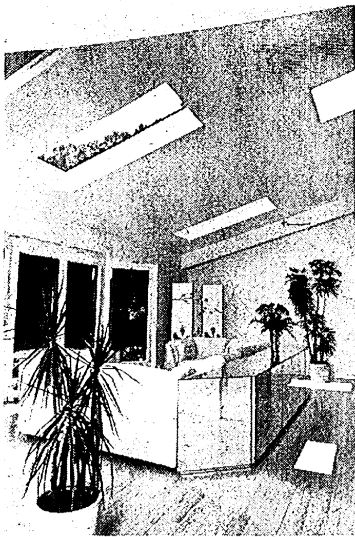
Two skylights set in tandem brighten and add excitement to this living room. Each skylight contains one-inch thick double pane glass installed in a lightweight aluminum frame, the interior of which is finished with California redwood.
