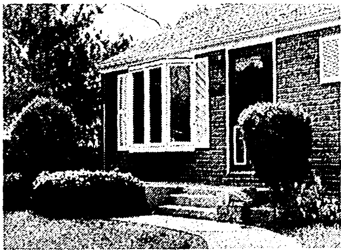
Enhancing the exterior appearance of this house, the bay window brings more light inside and conserves energy. All four sections of the thermalized, double glazed window open out for ventilation and easy cleaning
