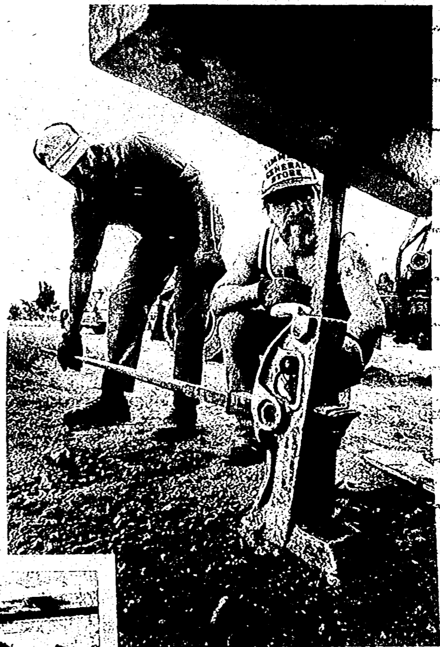
J.D. Porter (at left) sits on one of the skids under a house he is soon to pull along Wayne Road, his hand on part of the dolly that aids the work. Below, Gary Butler, like Porter, a Westland resident, struggles to change a flat tire on the trailer that holds a two-story brick house. At right, Al Edenton (left) and Butler use a railroad jack to lift a house.
