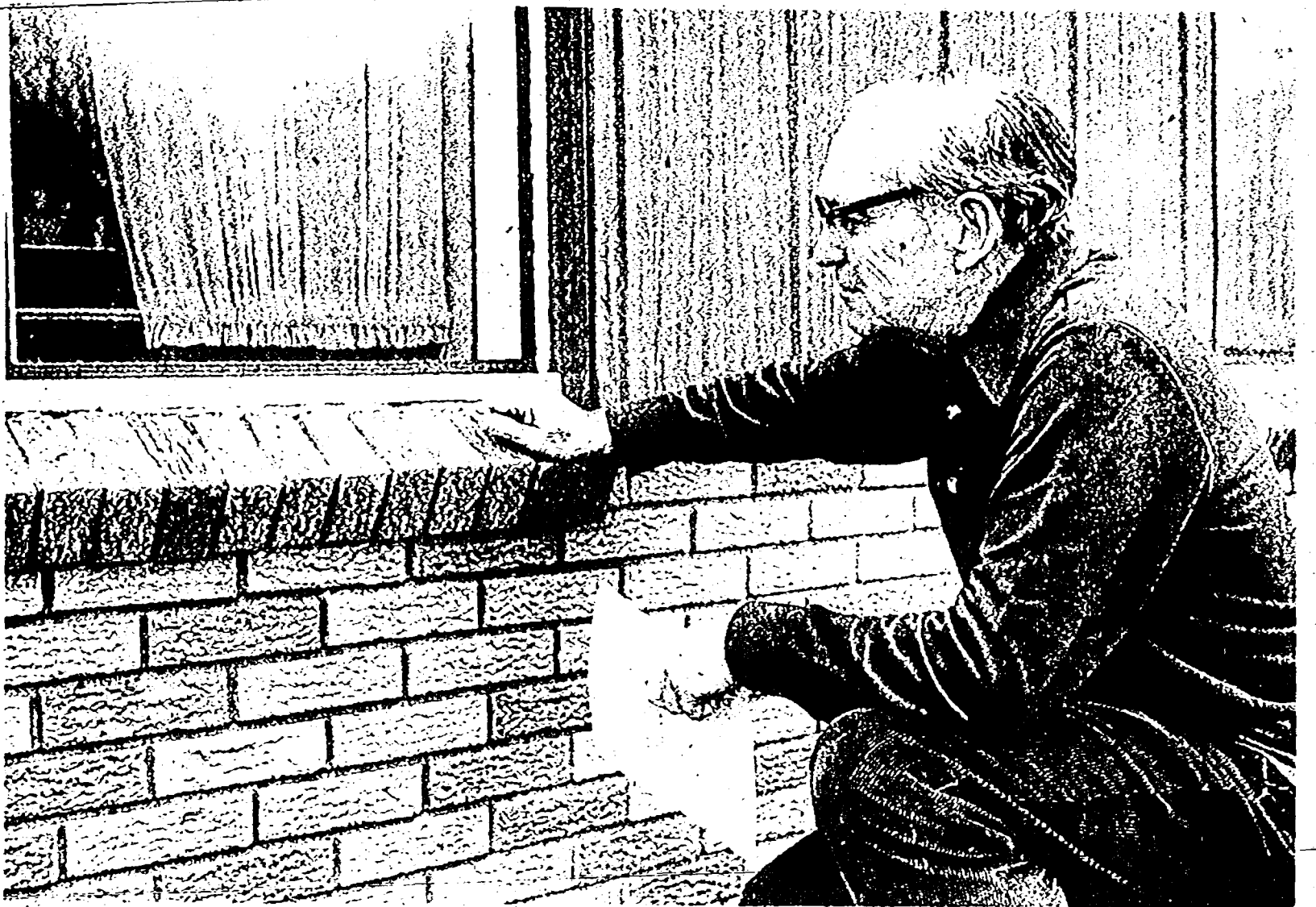
Energy analyst James Happ inspects caulking along the windows of the Westland Chamber of Commerce building on Ford Road.
