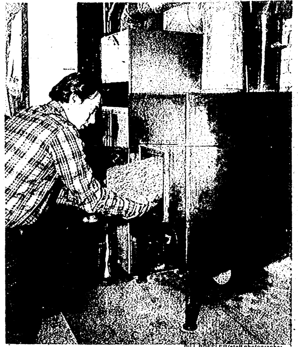
Mike Mangan loads up the stove he built at his Garden City home that uses his furnace blower system to circulate the heat.
