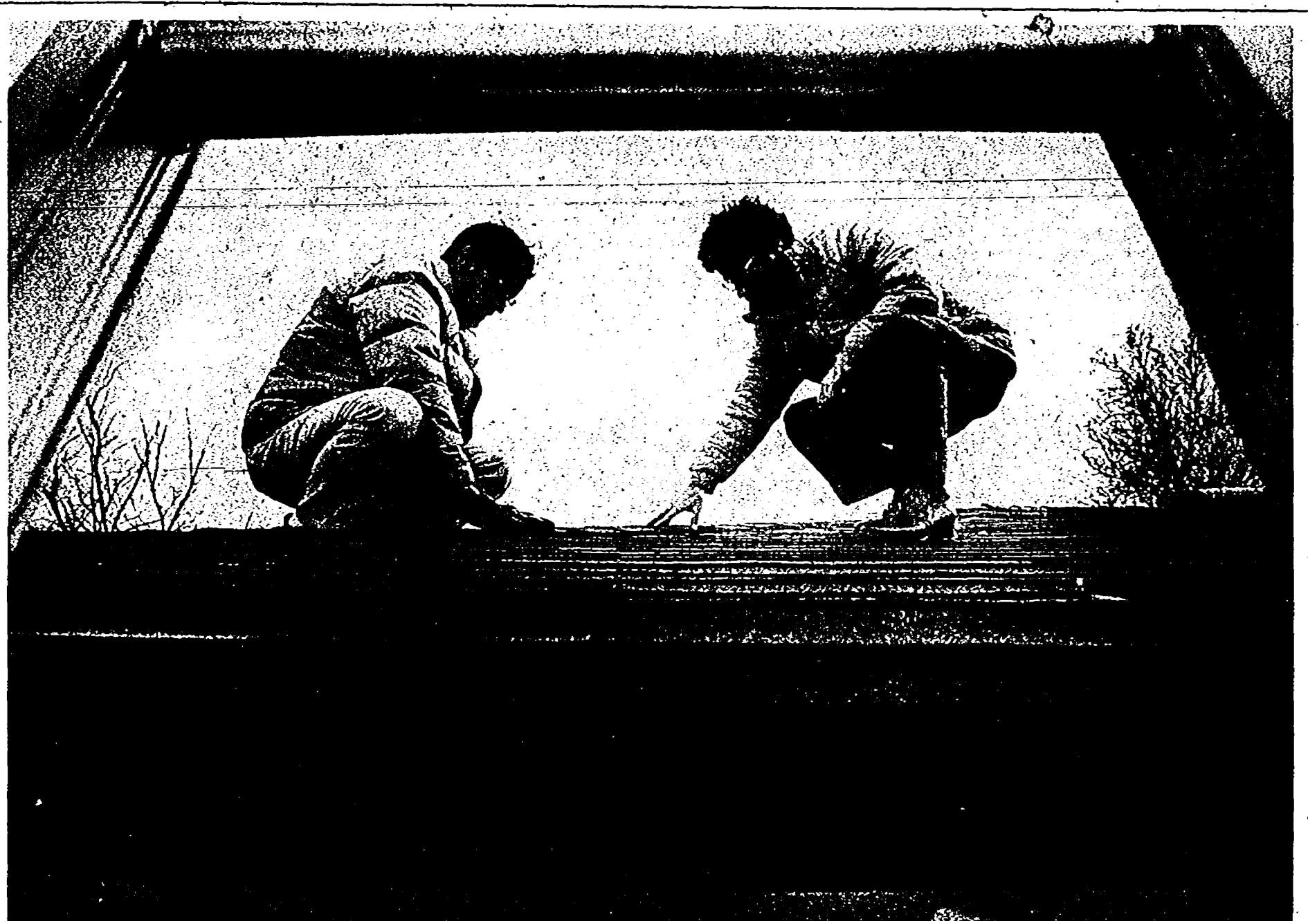
In their jobs with the neighborhood development program, Edward Gunther and James Gilbert have seen roofs with leaks so bad the floors were warped on the first floor of two-story homes.
